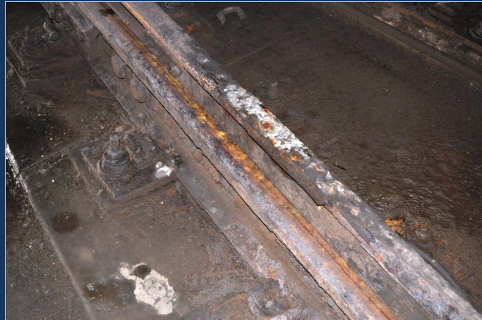
Corroded Running Rail
